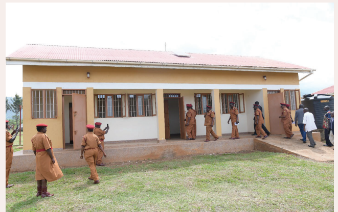
Newly constructed ward
