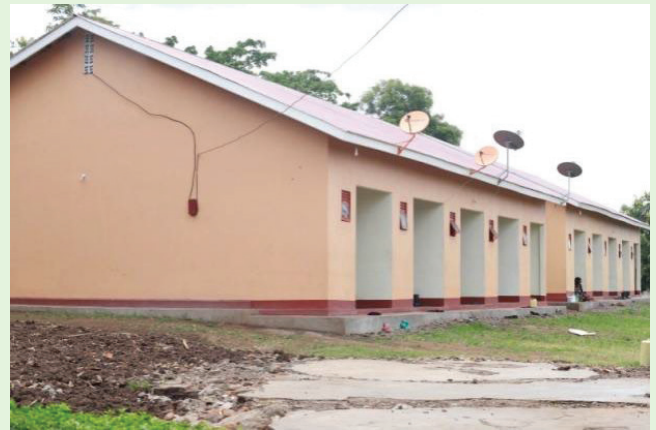
Newly Constructed Staff Houses at Ruimi Prison Farm in Western Region
